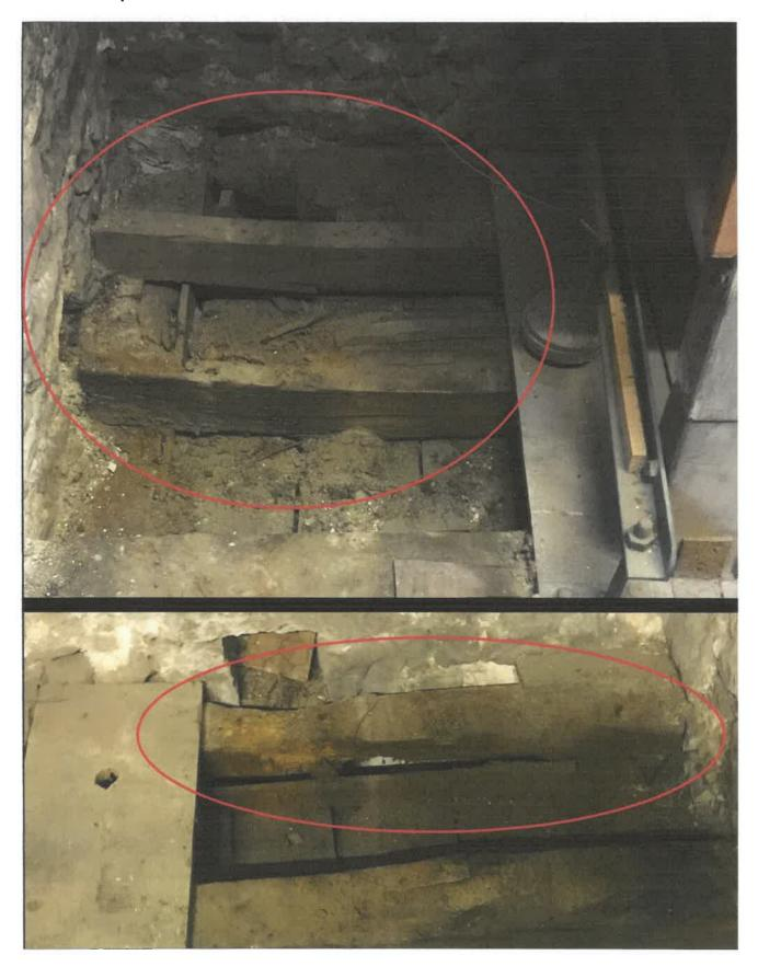
The towns historic clock and bells have been disconnected to prevent damage. The mechanism will need to be moved to undertake the beam and floor repairs.
